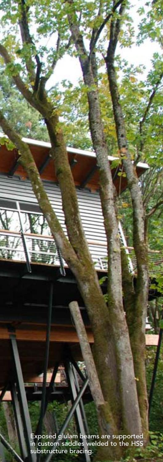
Exposed glulam beams are supported in custom saddles welded to the HSS substructure bracing.
